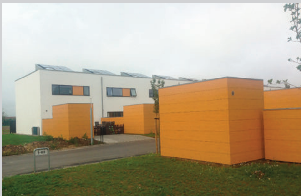
During 2012 60 low energy-housing units with prefabricated "Solar prisms" from VELUX and Danfoss was realised in Tranbjerg near Aarhus.
