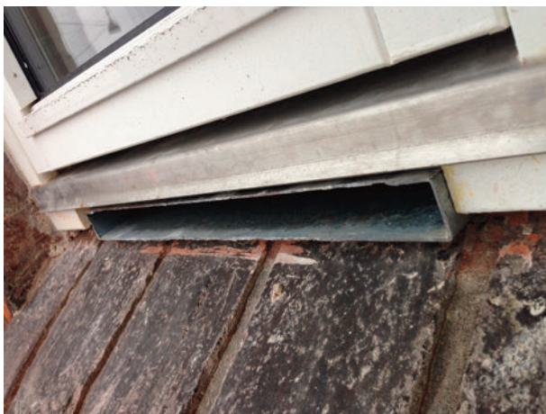
The new windows for the test apartment was supplied by the Danish EVD company with build in fresh air intake and used air exhaust integrated in the bottom of the window equal to \varnothing 140 mm.
