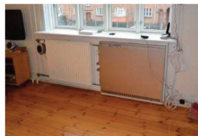
A very well-functioning example of window integrated heat recovery ventilation (HRV) was established at the P. Knudsens Gade housing area, administered by the housing association AKB, in Sydhavnen in Denmark situated in the Concerto area of the Green Solar Cities EU-Concerto project in Denmark.
