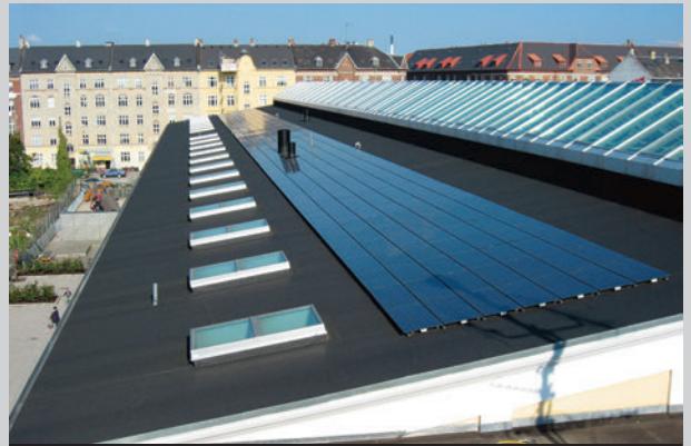
Valby School in Copenhagen with BIPV (Building Integrated Photo Voltaic).
