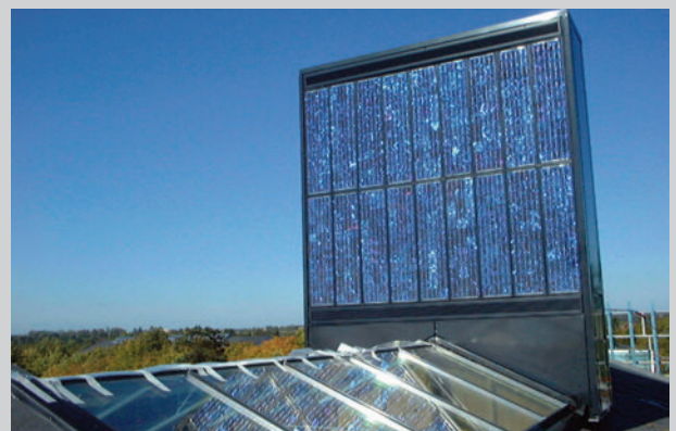
Solar chimney, Lundebjerg, Skovlunde was result of architectural competition with focus on PV and ventilation.
