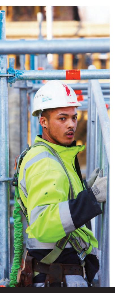
Sloping roofs require scaffolding to prevent people or materials falling from the edge. You must also fit edge protection to the eaves of any roof and on terraced properties to the rear, as well as the front. Where work is of short duration, (tasks measured in minutes), properly secured ladders to access the roof and proper roof ladders may be used.
