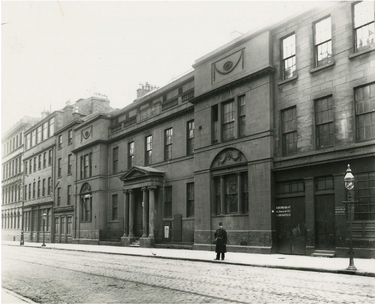
Photograph 1902, shortly before demolition. Original building 1831.
