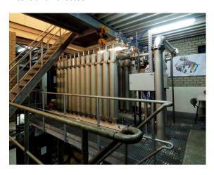
**Figure 2.** Picture of the ceramic membrane filtration demonstration plant at Vitens production location, Wierden, NL
