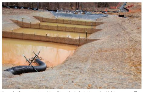
Example of a construction site sediment basin featuring a piped inlet, porous baffles, and a skimmer outlet
