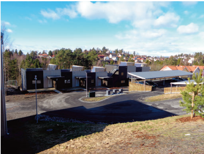
Roofs consisting of Aventa Solar Thermal collectors
