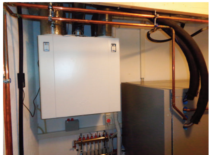
Heat recovery ventilation system
