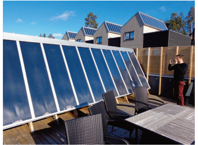
Roof terrace with approx. 14m 2 Aventa Solar Thermal collector. This technology has a far better yearly COP (coefficient of performance) than outdoor air heat pumps
