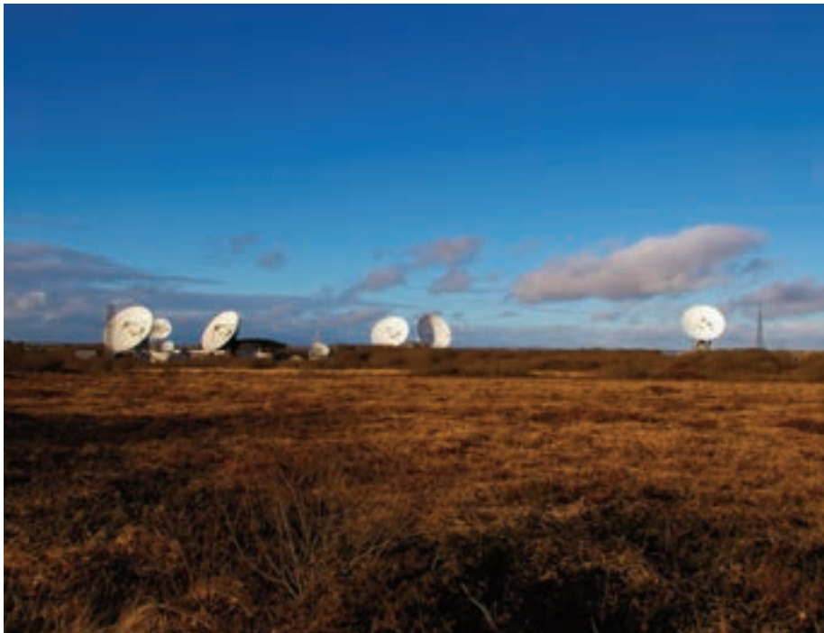
Goonhilly Earth Station where a similar conversion of ex-telecommunications antennas into radio telescopes is ongoing in partnership between UK universities and the SME GES Ltd
