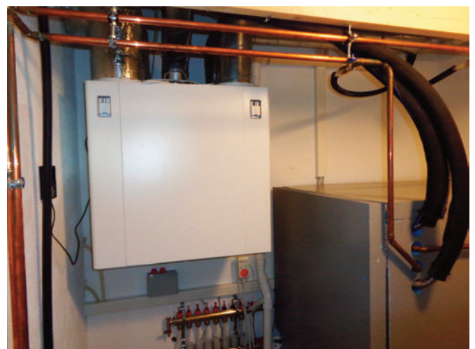
Heat recovery ventilation system
