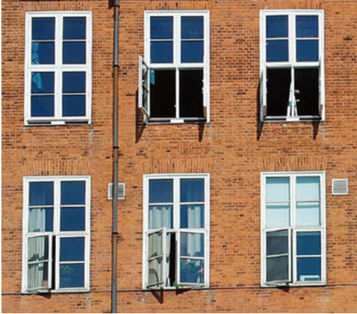
New windows with integrated fresh air intakes and exhaust outlet in window frame
