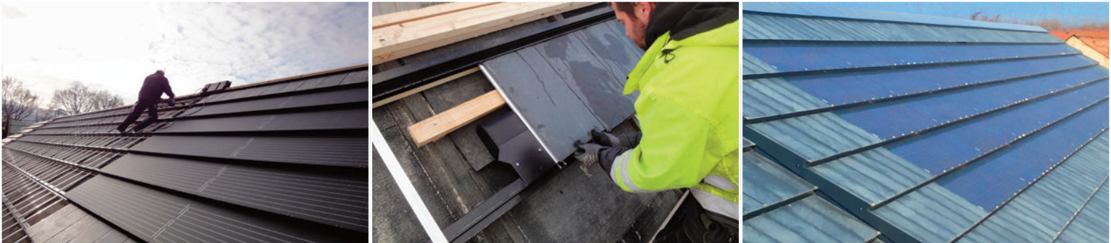
Fig 1. A newly developed "Complete Cover" roof from Komproment in Denmark. It includes a build-in possibility for placing exhaust air armatures, avoiding shadow problems from normal types of exhaust air armatures, and this is with a proven operation quality according to tests at Aalborg University in Denmark
