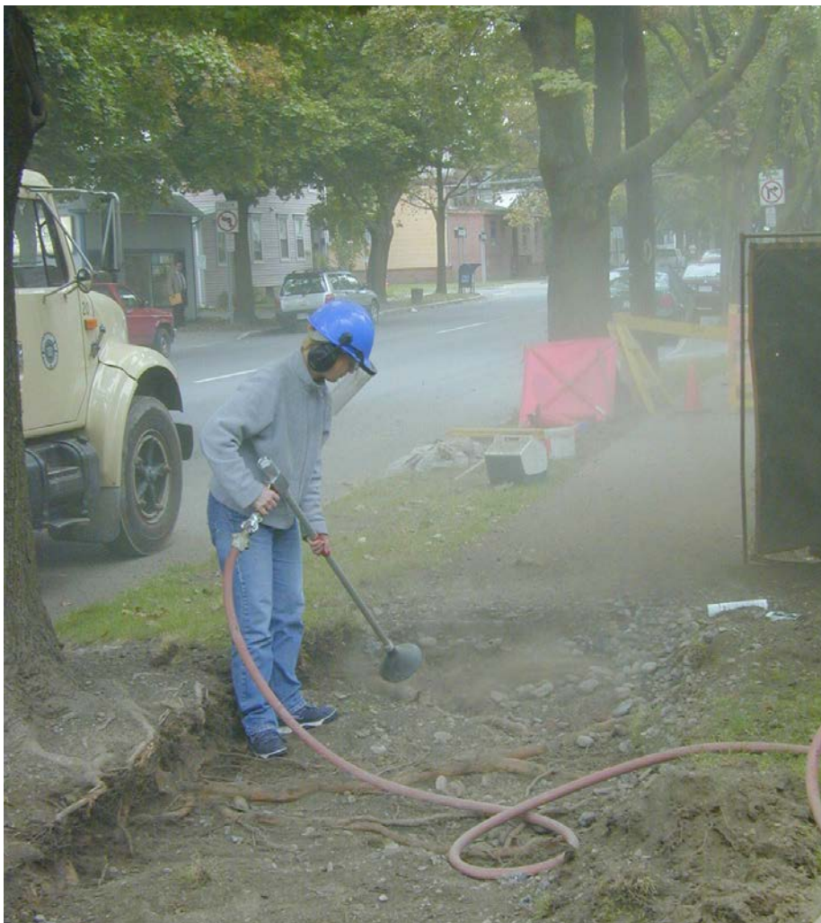
Using air excavation tools we uncover roots
