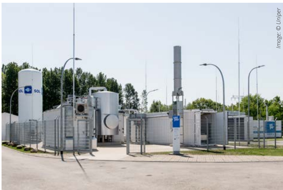
One of STORE&GO's three demo sites: Methanation demo plant in Falkenhagen, Germany, with the rounded methanation reactor at the centre (© Uniper)
