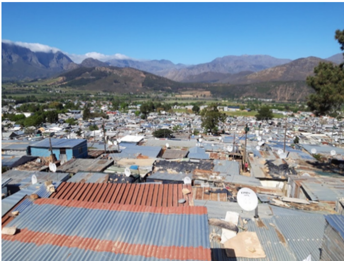
A rapidly expanding informal settlement overlooking vineyards and wineries in the Franschhoek valley (80km east of Cape Town)
