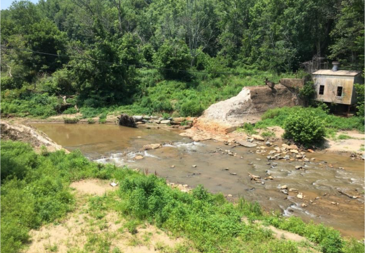
Figure 1 – Removal of a Low-Head Power Dam. The legacy sediments behind this structure have been distributed throughout the stream bed up to 50 km downstream.
