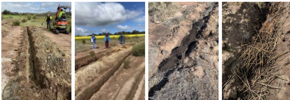
FIGURE 2. a and b. Drilling the permeable biomass walls, c. walls filled with organic materials, including biochar, and d. wall filled with organic materials, including straw.
