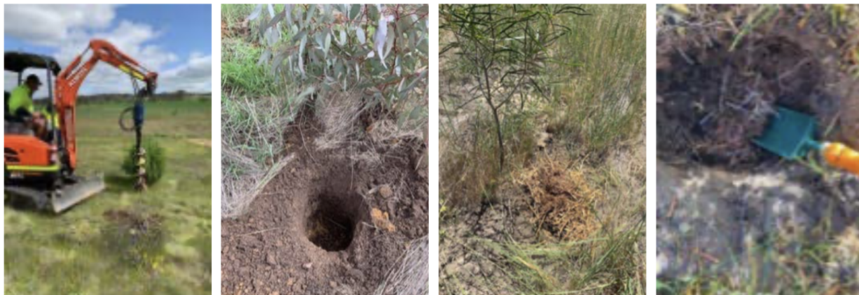
FIGURE 1. a. Drilling of the permeable biomass wells, b. new well before application of organic materials, c. well filled with organic materials adjacent to a tree, and d. The contents of a well after several months show that roots have penetrated the organic materials.
