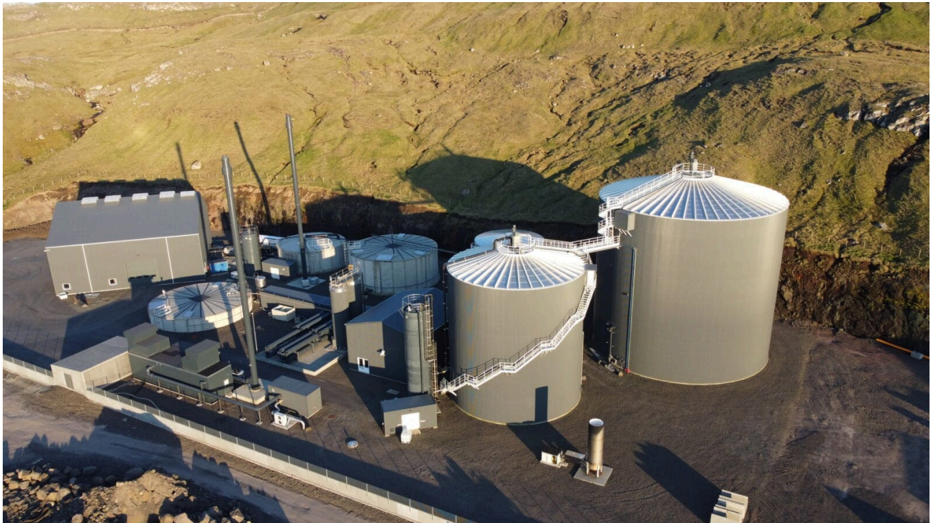
Figure 4: The FÖRKA biogas facility in the Faroe Islands has the capacity to process up to 100,000 tonnes of organic waste annually. One of Terraforming LIFE's partners, SMJ, led the design of that plant and will use the experience gained there as the foundation for developing the biogas plant planned for Iceland. The figure is from SMJ's website.
